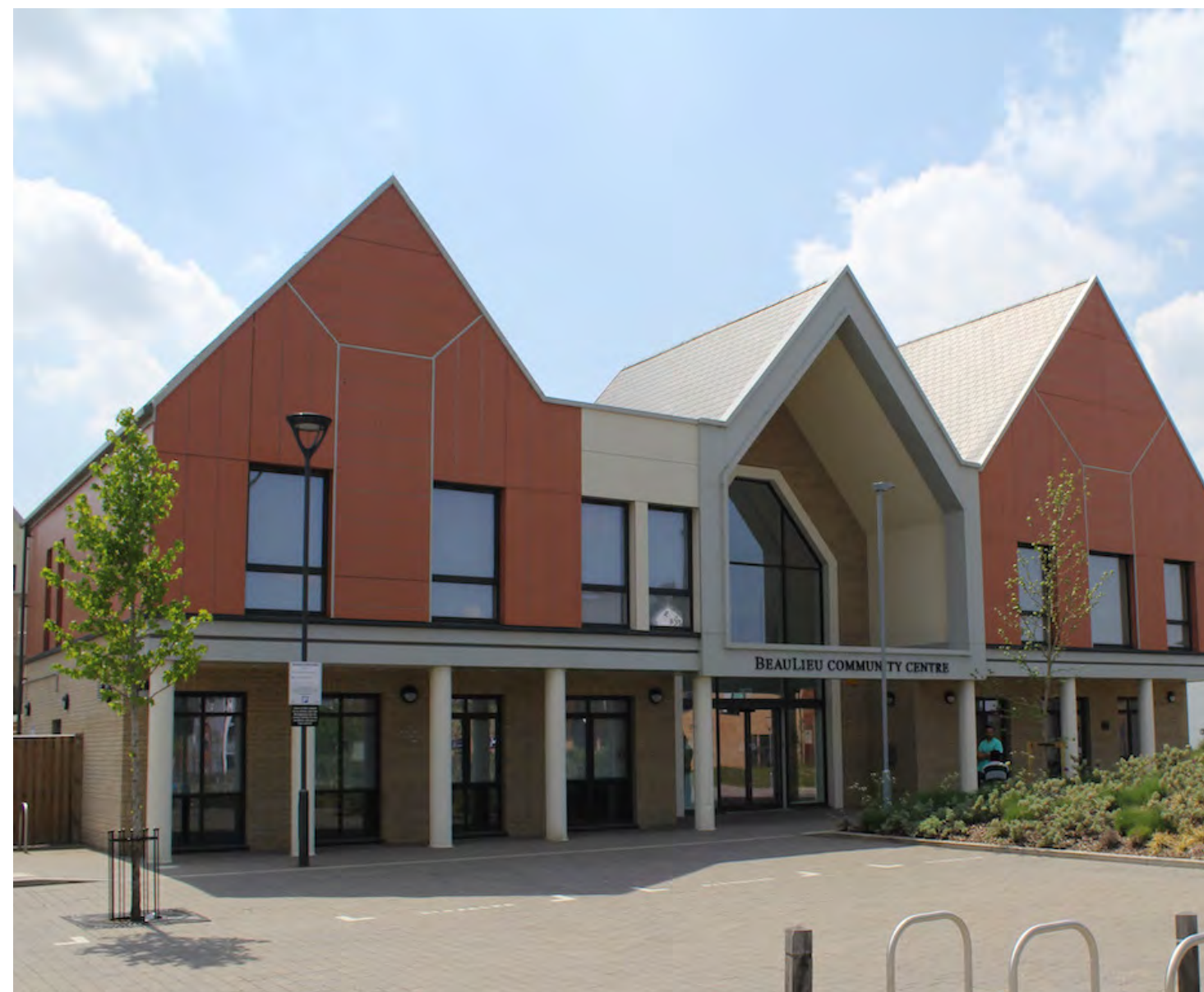
▲ A Community Hall could link to a civic space at the school and Dell Spring, creating a central Hub
