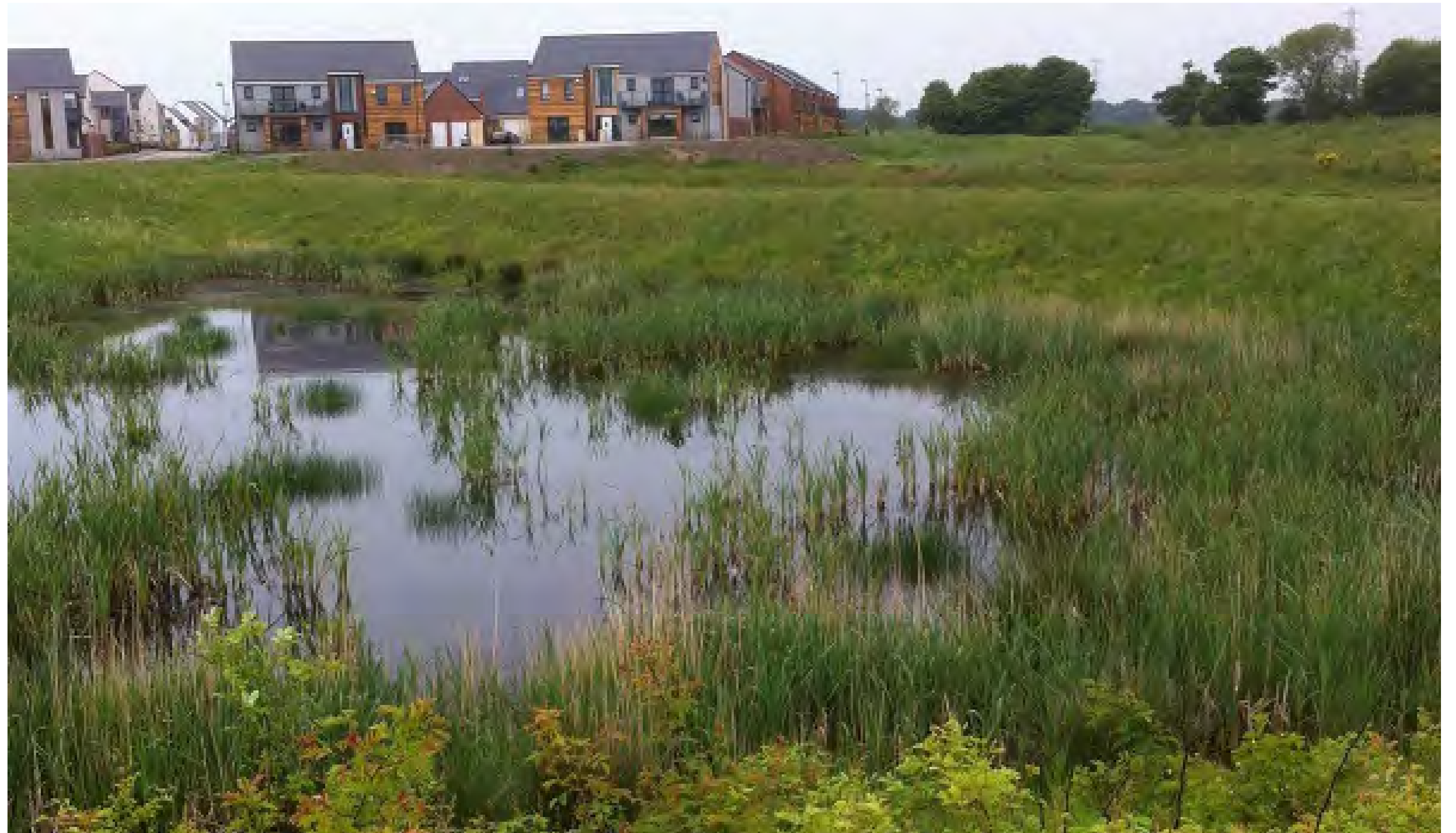
▲ The drainage basins are expected to be dry the vast majority of the time, and should be overlooked by the new homes to provide passive surveillance and to create attractive open spaces
