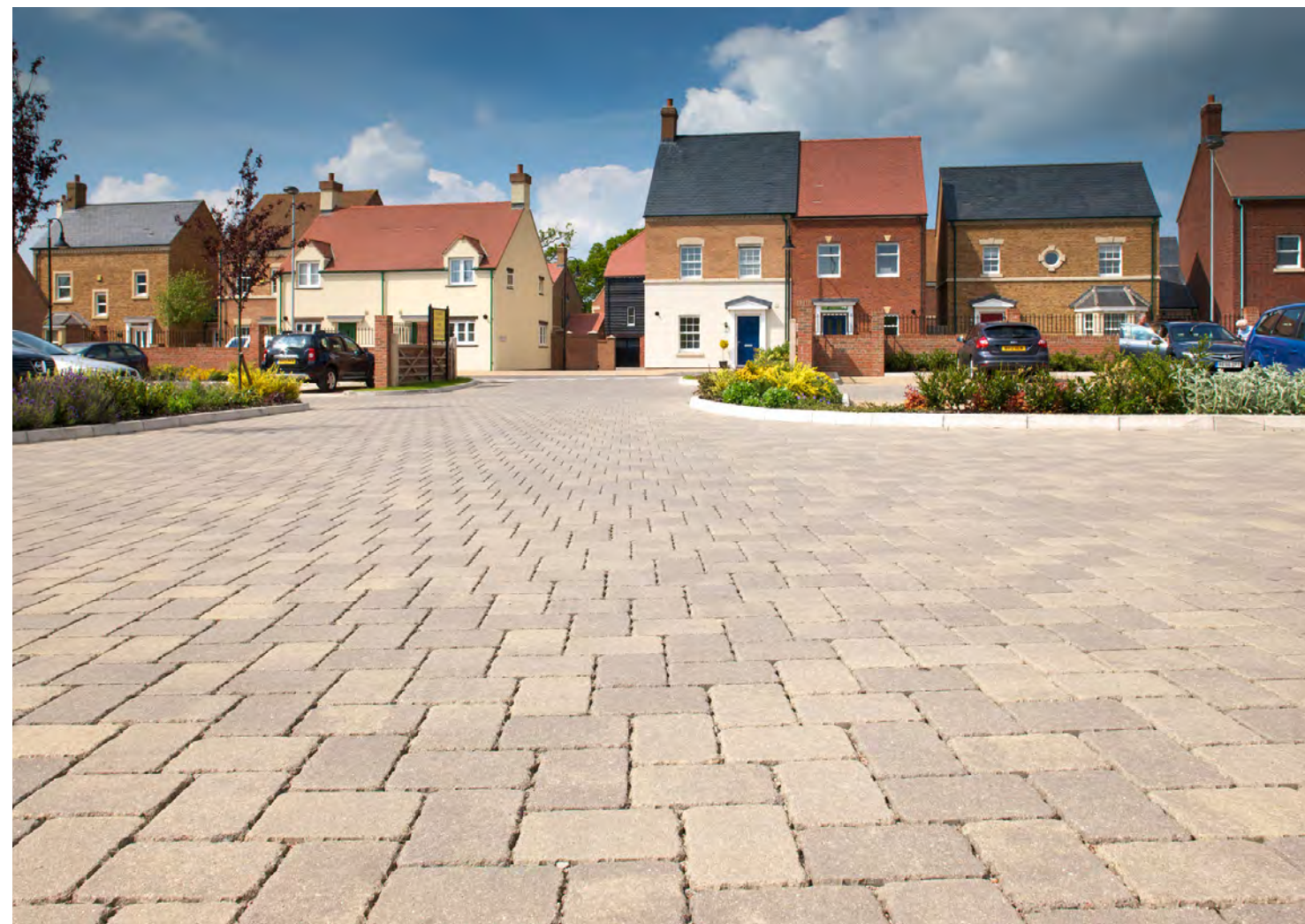
▲ The use of block paving on roads can help slow traffic speeds
