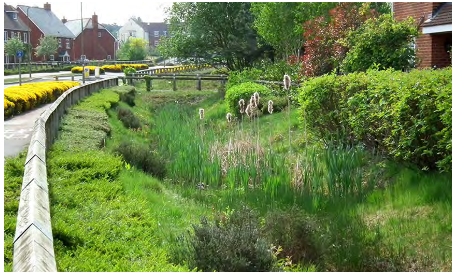
▲ Swales could be planted with suitable vegetation to create attractive landscape elements which benefit ecology and condition the surface water run-off
