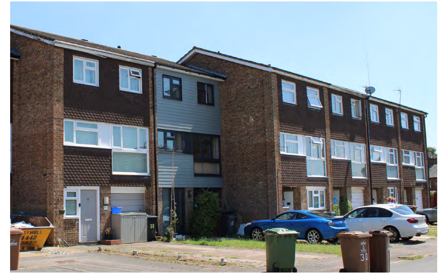
▲ Much of the architecture in Stevenage is reflective of the era in which it was built
