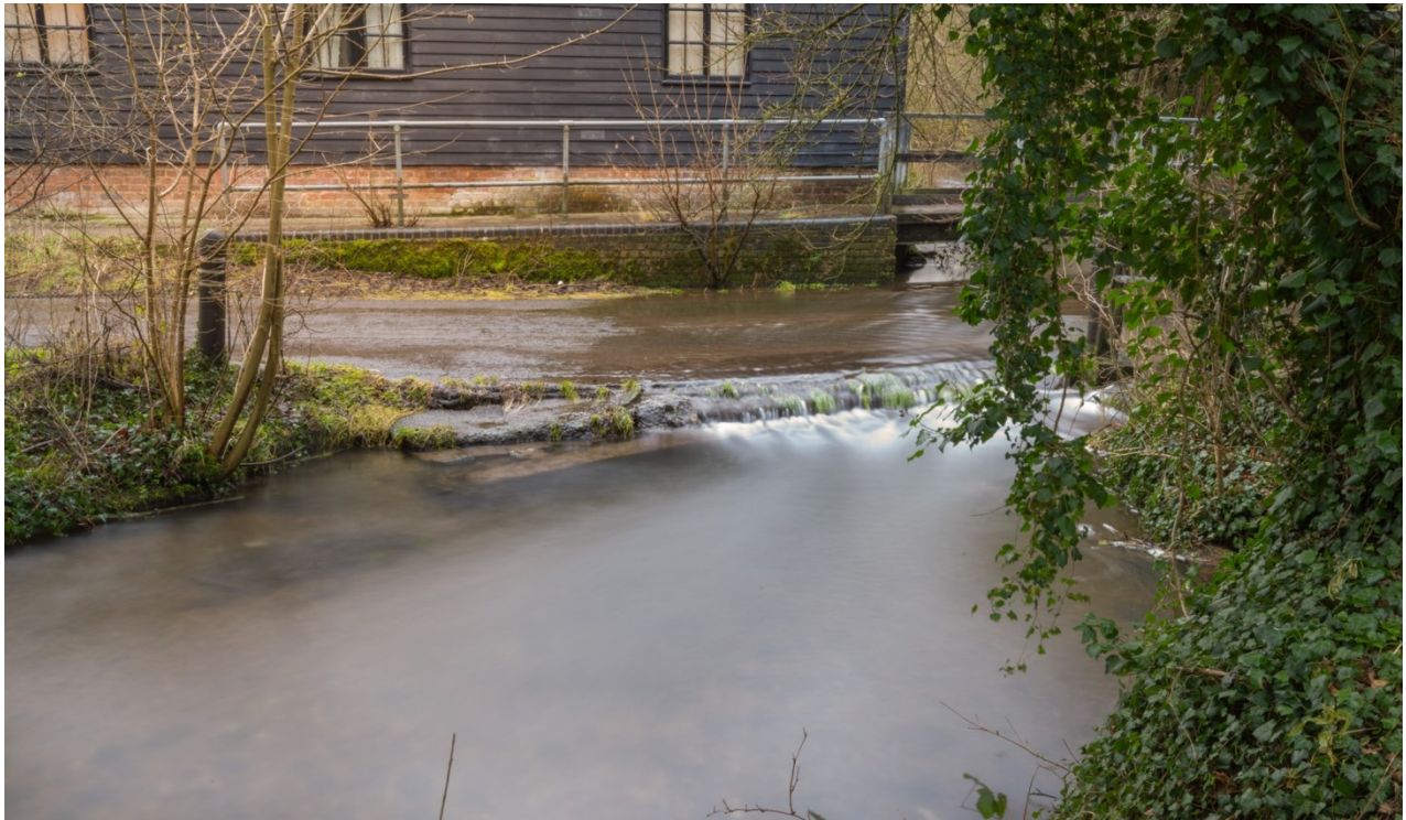
Figure 52: Cart Ramp near Fulling Mill
