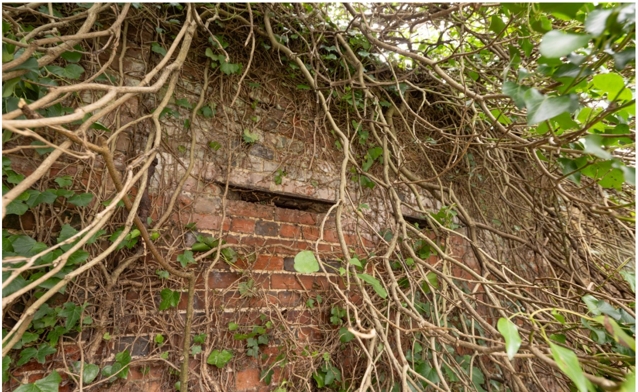
Figure 49: Gun Slit in wall, High Street
