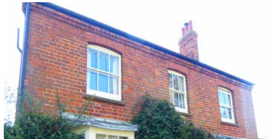
Figure 58: Example of brickwork used for walls and timber sash windows
