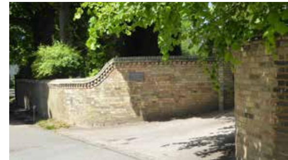
Figure 46: Boundary wall, Springhead
