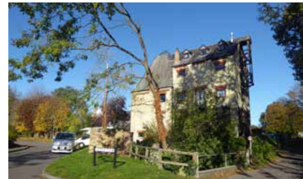
Figure 44: Former Brewery Building, Fordham Close
