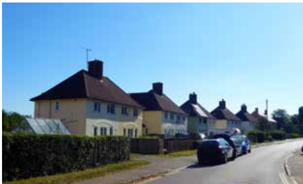
Figure 54: Station Road, looking north
