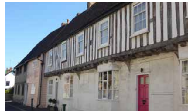
Figure 23: 57, 59 and 61 High Street
