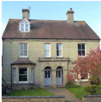
Figure 27: 86 and 88 High Street
