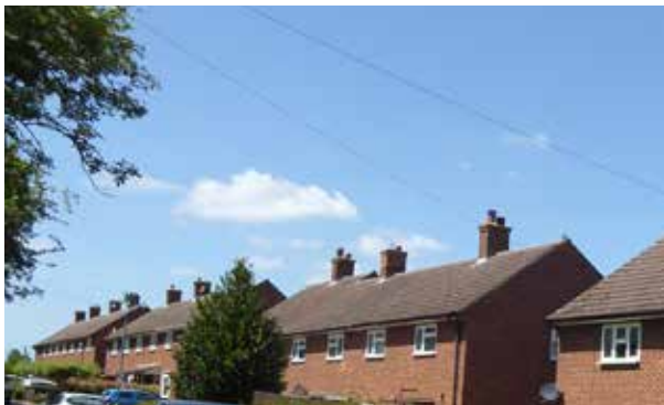
Figure 66: Brown plain tiled roofs within the Character Area
